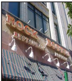
Externally illuminated sign using gooseneck lamps
